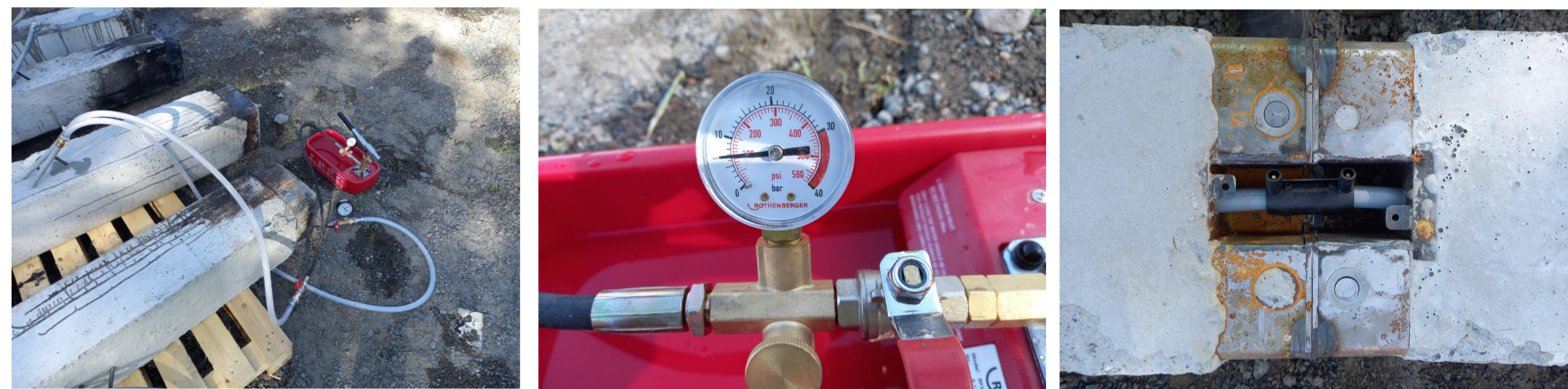
Fig. 5. Hydraulic pressure test
