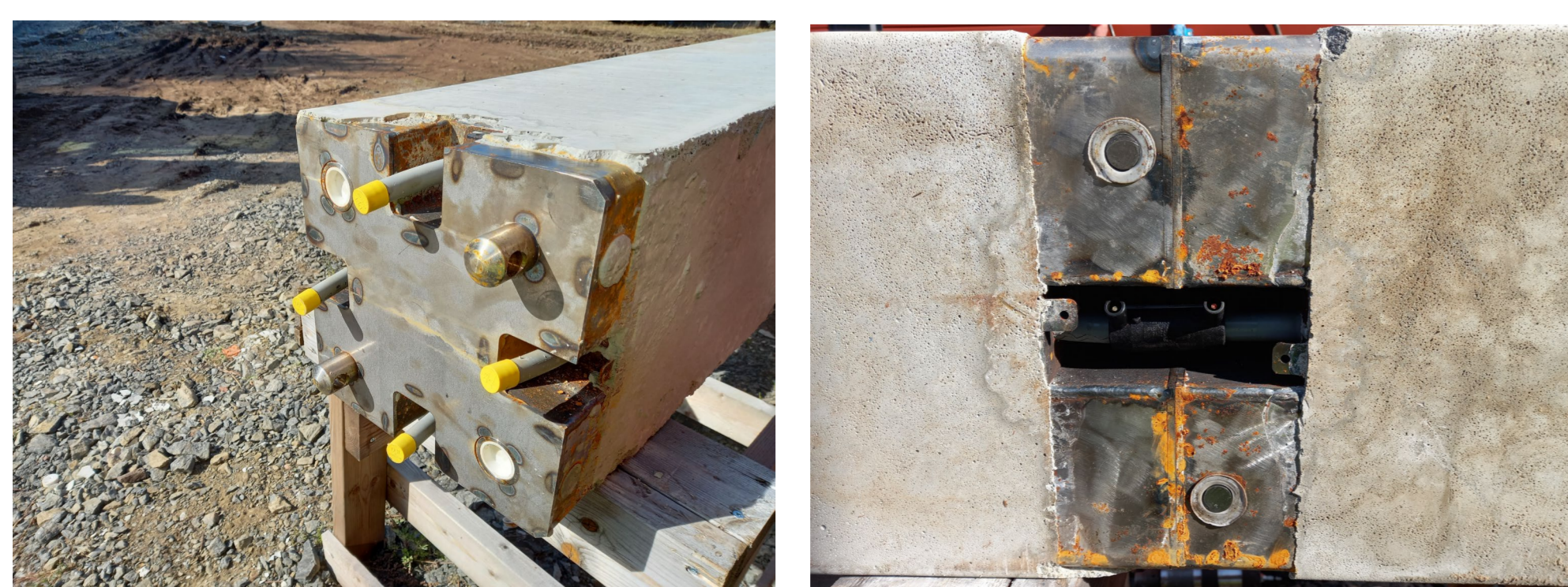
Fig. 3. Connection and coupling of joints and HE pipes
