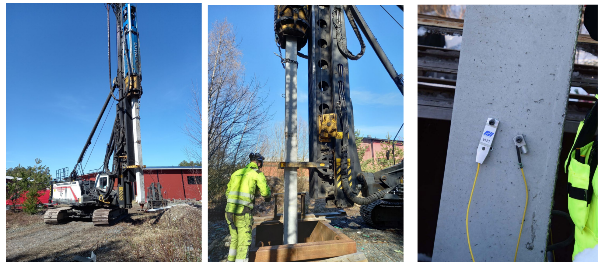
Fig. 4. Impact test with PDA measurements
