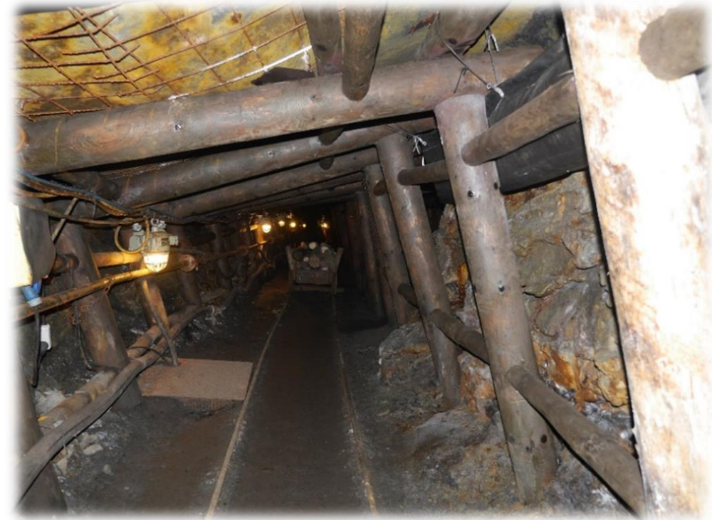
Nightingale visitation colliery in Witten, Germany (wooden beam construction)
