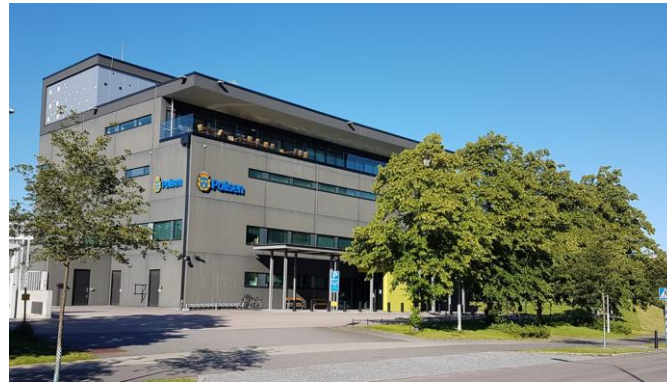
Polishuset, Malmö (2012) 12 boreholes, 200-m deep each
