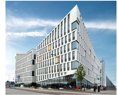
Klipporna, Malmö (2014) 70 boreholes, 220-m deep each
