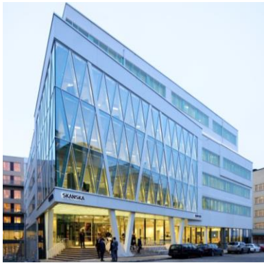
Entré Lindhagen, Stockholm (2013) 144 boreholes, 230-m deep each
