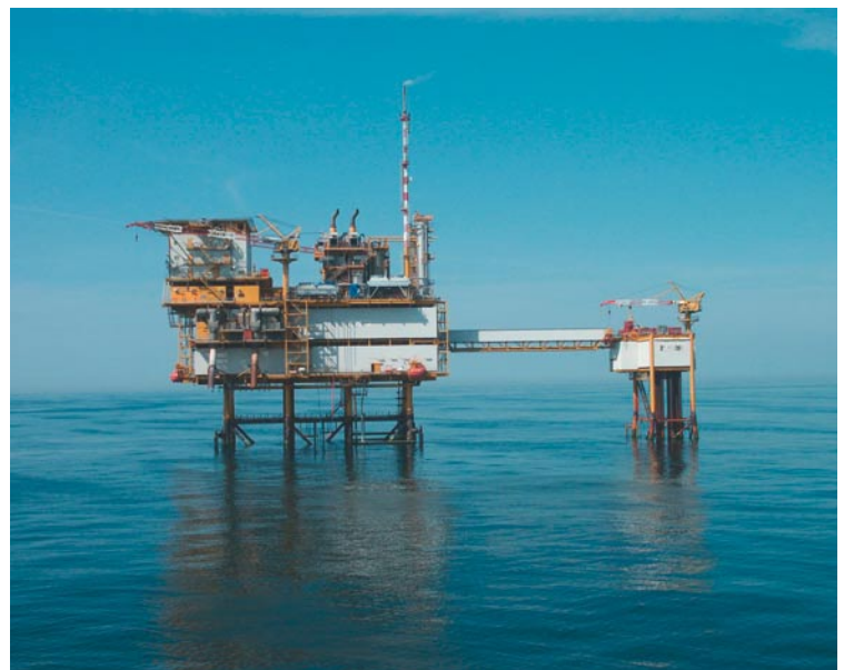
Fig 2: The K12-b platform consists of a well-satellite on the right hand side, connected by a bridge to the gas treatment platform on the left. The treatment platform shows on the top structure, the accommodations quarters on the left and the upper part of the CO 2 treatment columns on the right. (Courtesy Gaz de France)
